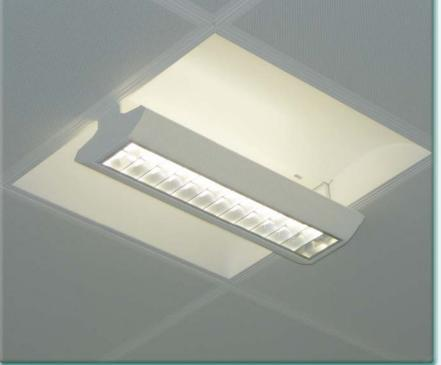
Some floors of this building were to be occupied by a known tenant yet others were fitted out to be let. In the absence of being able to discuss specific requirements the client realised the benefit of using our patented RET Adjust - Whilst marketing the floors all fittings were installed with the gondola recessed yet if required could be easily dropped to meet LG7, thus helping with marketability and compliance.
